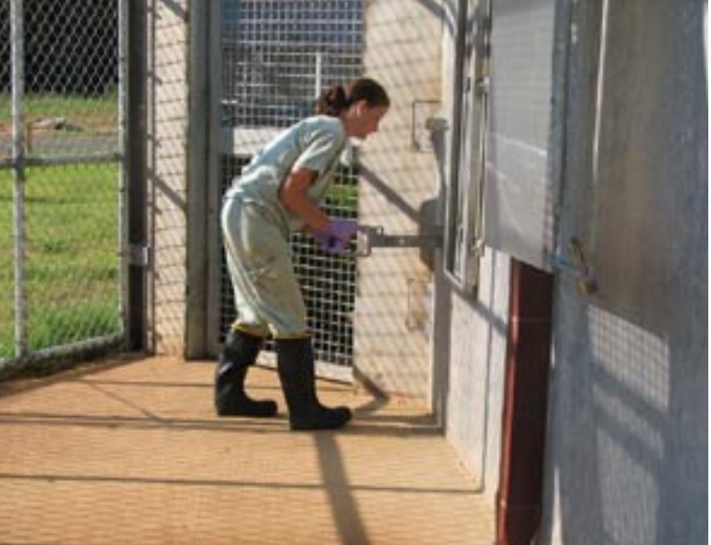
Manual slider doors made of polypropylene slide easily. View ports are provided for keepers to see both sides of each door.
