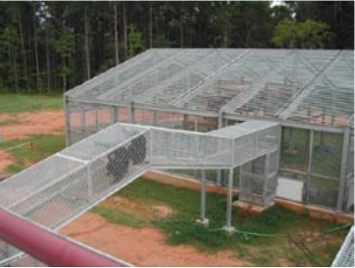
Twin overhead transfer chutes connect holding building to habitat feeding shelter (left) and the "jungle gym" (right).
